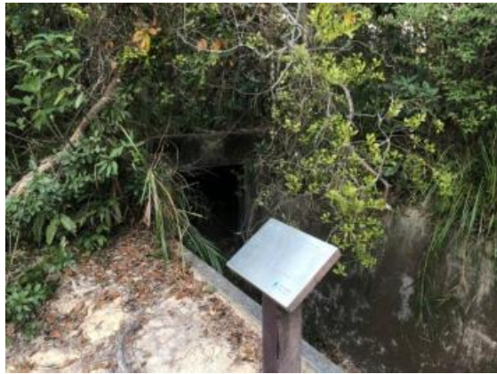
Fig. 5. Disrepair of the Redoubt Relic Tunnel with Overgrown Vegetation and Graffiti Damage
