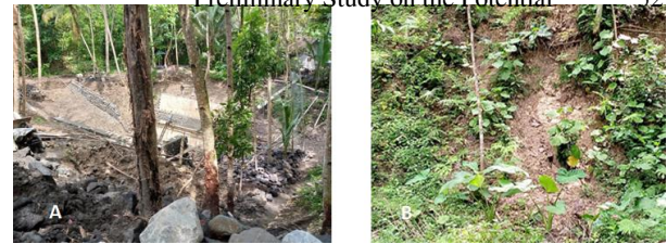
Figure 9. A) Location of the mining cave entrance being renovated; B) The outcrop condition of the Sentolo Formation is strongly weathered.
