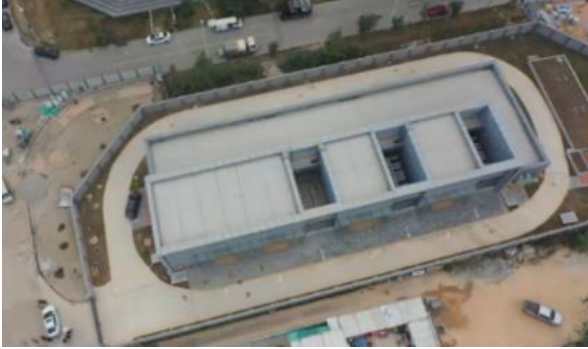
Fig. 1. View of substation.
