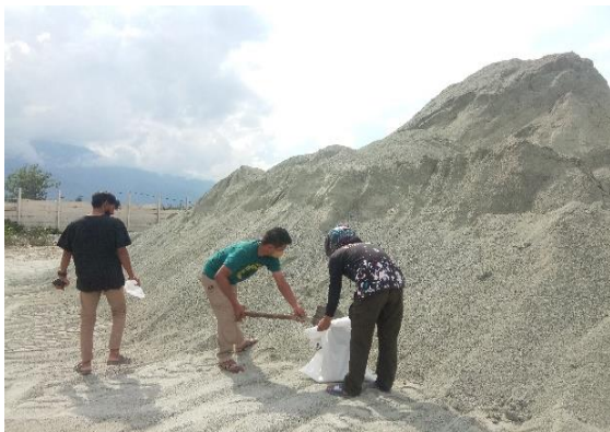
Fig.2. Aggregate Material Pick-Up
