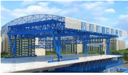
(a). Opening status of rigid telescopic shed
