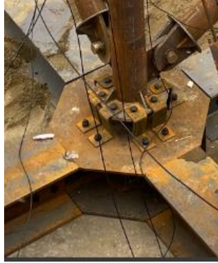
Fig. 3. Bolt connection method for modular shed.
