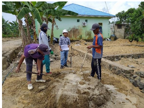
Fig 10. Manual mixing of concrete
