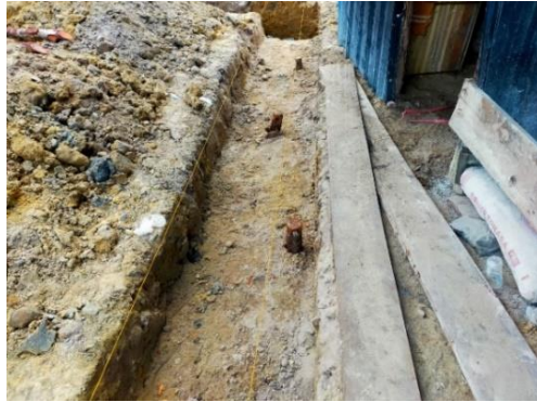
Fig 7. Continuous stone foundation with mangrove stakes
