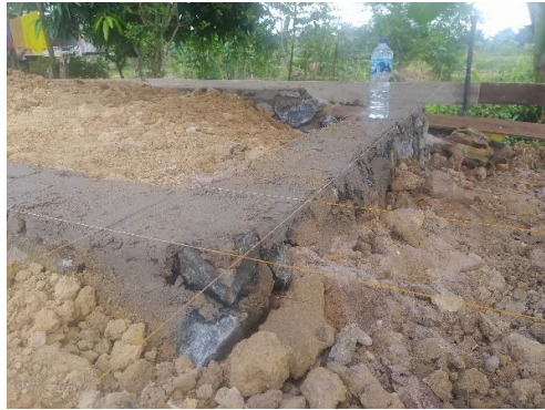
Fig 4. The house construction stage has been designed symmetrically.
