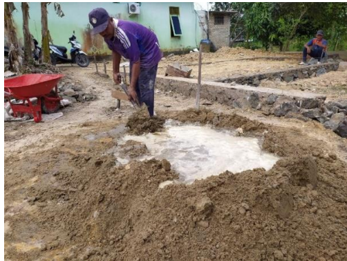
Fig 6. Use of mortar with 1pc specs: 4 sand
