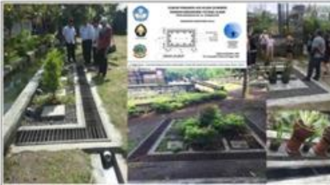
Fig 6. Final view of Rainwater Harvesting Wells types 1, 2, and 3 with various forms of placement according to available land.
