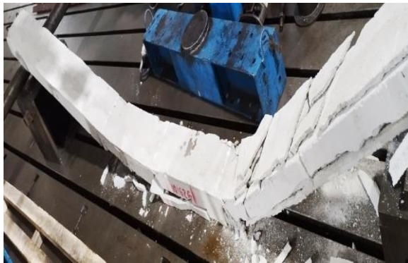
Fig .4. The collapse of the beam
