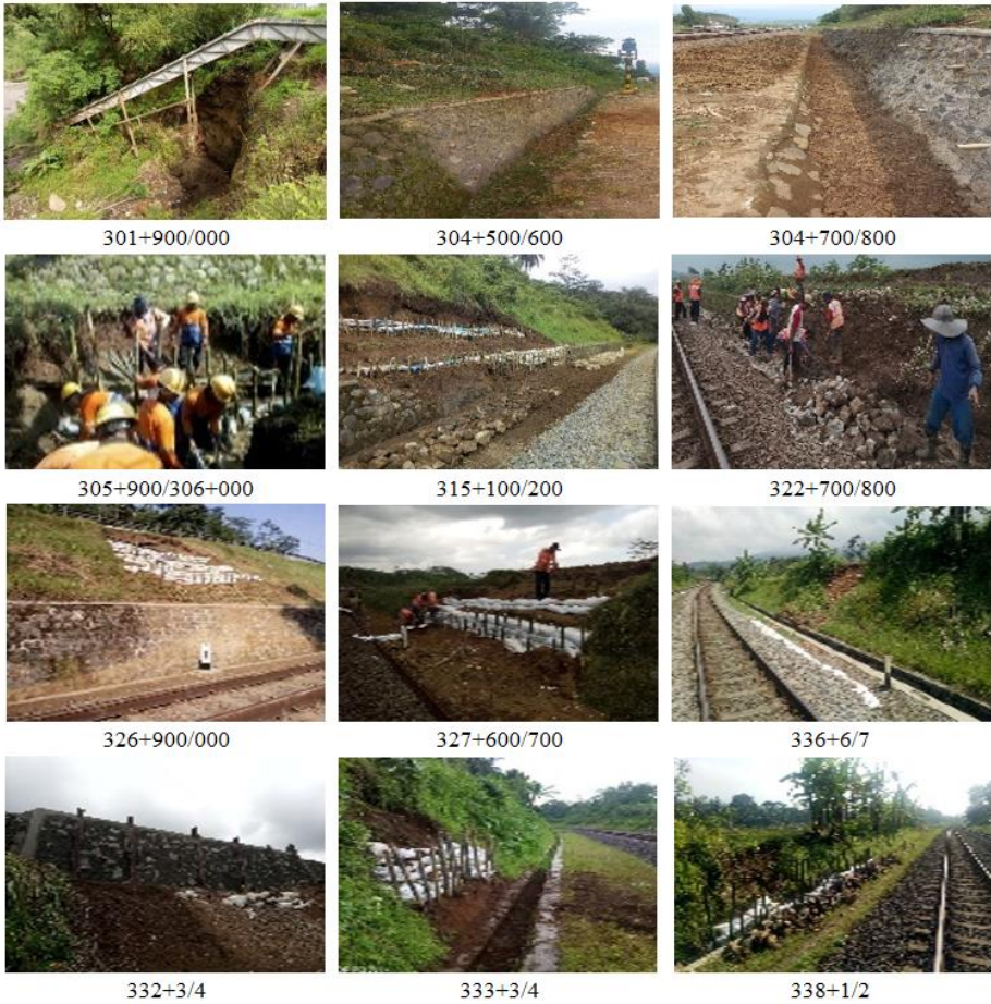
Fig. 3. Documentation of Reinforcement for Landslide Events
