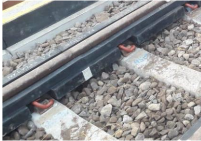
Fig. 2. Concrete level crossing fastener
