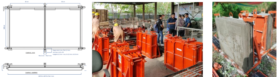
Fig. 4. Mold for the wall panel components of the Puzzle Polsri house. Source: Author, 2023
