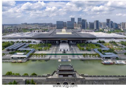
Fig. 4. Aerial view of Suzhou Railway Station
