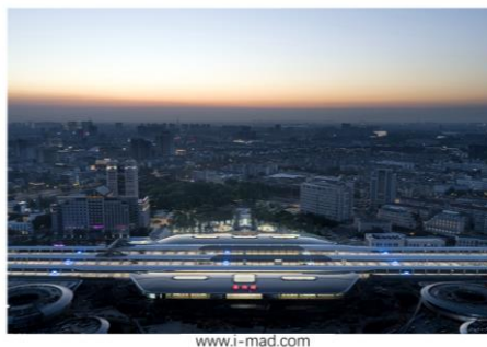
Fig. 5. Aerial view of Jiaxing Railway Station;
