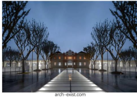
Fig. 7. Jiaxing Railway Station: new and old station building.
