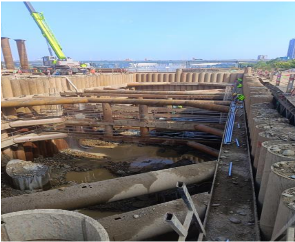
Fig. 6. Construction Scene of the Cofferdam
