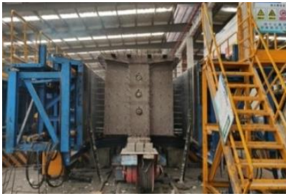
(a) lateral installation of hydraulic side formwork
