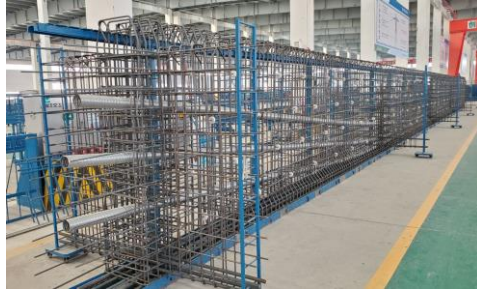
T-beam web reinforcement skeleton tying by unit frame
