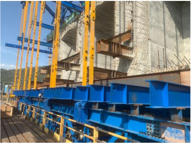
Fig. 4. Reaction frame for preloading.
