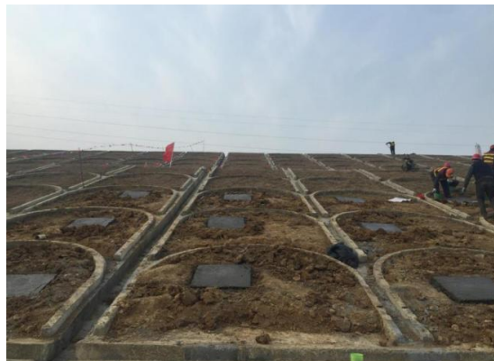
Fig. 14. Site after pile-anchor joint reinforcement
