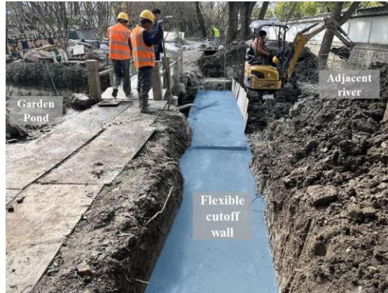
Fig. 6. Flexible cutoff wall construction
