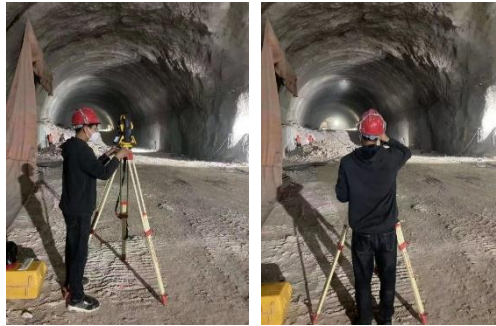
Fig. 2. Surrounding rock deformation monitoring.
