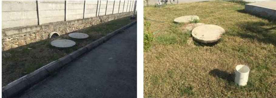
Figure 3. Rainwater management using infiltration wells.
