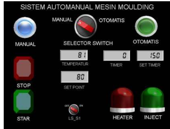
Fig 10. HMI heater and temperature OFF
