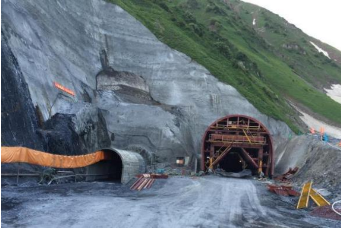
(b) Tunnel entrance
