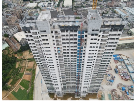
Fig. 6. Building after Disassembled all Aluminium Formwork (Source: Author)
