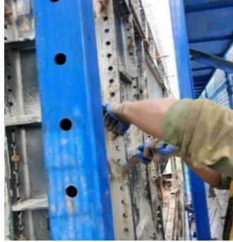
Fig. 2. Aluminium Alloy Formwork Installation (Source: Author)
