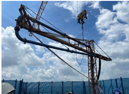
Fig. 3. Pouring Concrete by using concrete pump (Source: Author)
