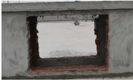
Fig. 5. Then open the electromechanical hole
