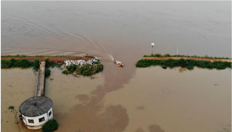
Fig. 1. Site of embankment breach
