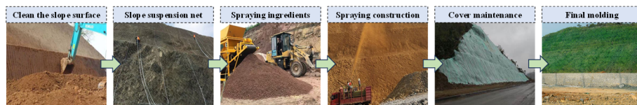
Fig. 2. Spray sowing techniques for ecological slopes
