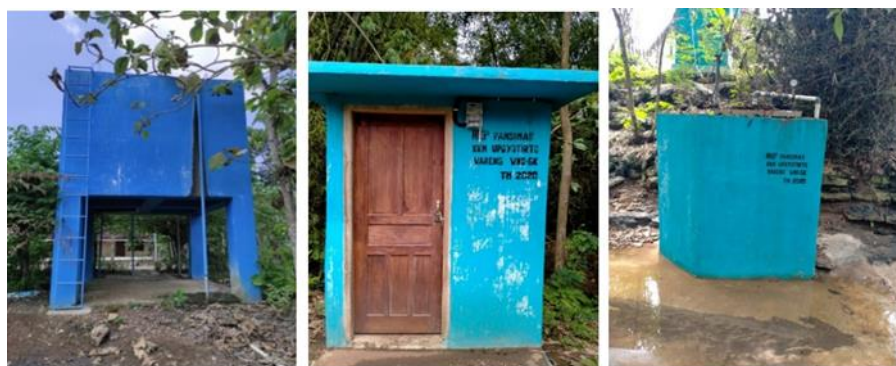
Fig. 1. Infrastructure for Providing Drinking Water and Sanitation in Wareng Village
