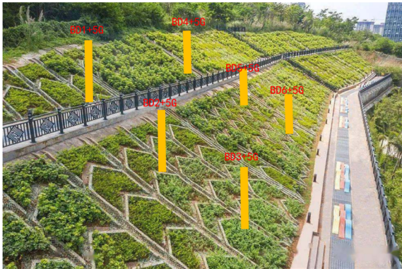
Fig. 5. Schematic diagram of slope displacement monitoring points
