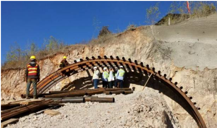
Fig. 1. Diagram of Advanced Long Pipe Shed
