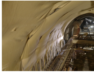
Fig. 2. On-site construction of laying and hanging geotextiles
