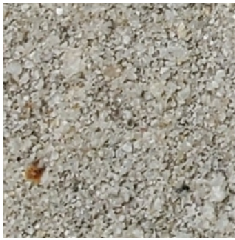
(a) Concrete background image
