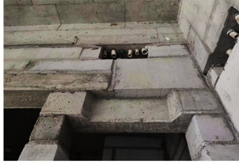
Fig. 5. Prefabricated notched over beam installation
