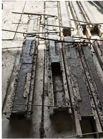
Fig. 4. Concrete pouring and forming of notched over beams
