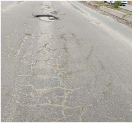
Fig. 1. Rutting of pavement along the length.
