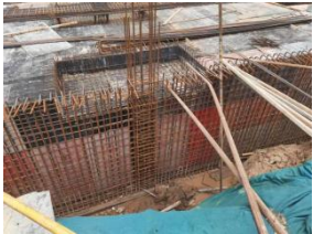
Fig. 2. On site foundation (Image source: Photo taken on site)
