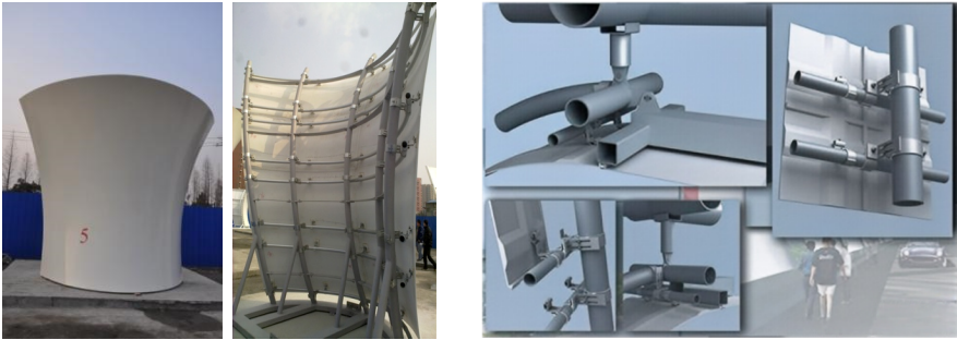
Fig. 7. FRP material scheme and technical implementation of hyperboloid surface of large special-shaped columns in Hangzhou East Railway Station
