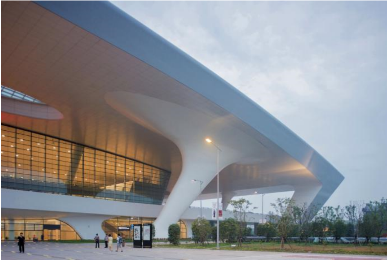
Fig. 2. Hyperboloid special-shaped columns and corner columns at the west entrance of Hangzhou East Railway Station Building
