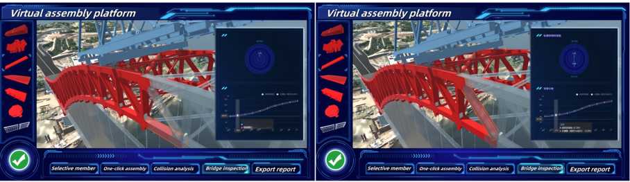
Fig. 9. Installation of the lower chord member for B21B22 segment and installation of the diagonal member for A21C22 segment
