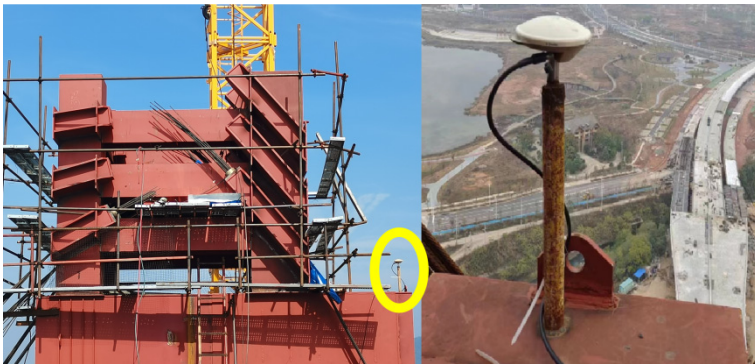
Fig. 3. Schematic diagram of real-time monitoring points for anchor tower
