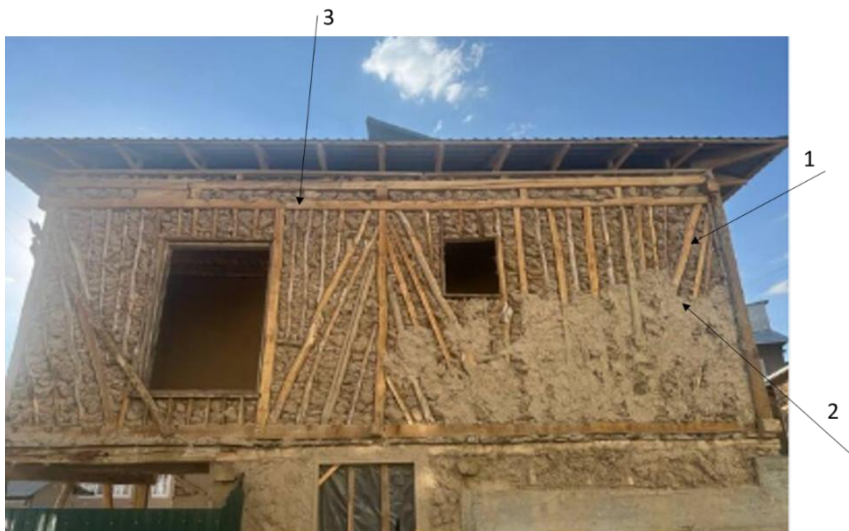
1- brace beam, 2- adobe 3- frame strapping beam
