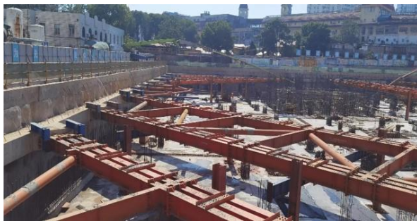
Fig. 4. Schematic diagram of horizontal support enclosure structure
