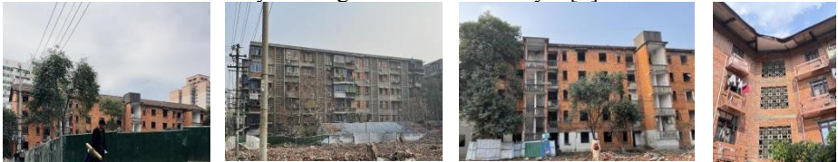
Fig. 1. Destruction of Soviet-style red-brick buildings in Caojia Alley Lane.
