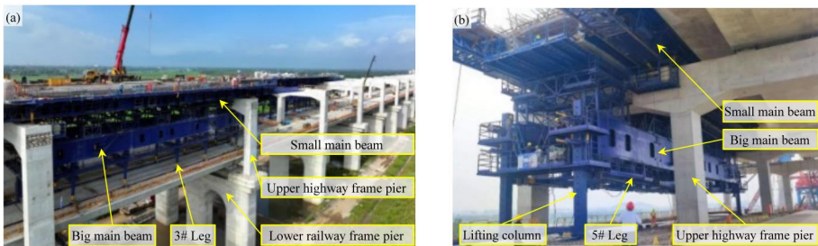
Fig. 3. Pictures of the new split movable scaffolding system during construction: (a) casting condition; (b) hole passing condition.
