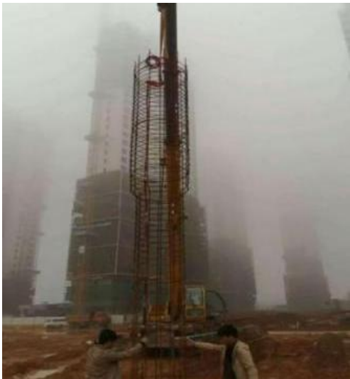
Fig. 2. Construction of stepped pile.
