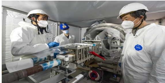
Fig. 5. Joint assembly on site [9]
