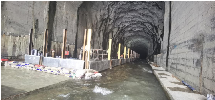
Fig. 10. Actual picture of the tunnel entrance and the outside of the cofferdam.
