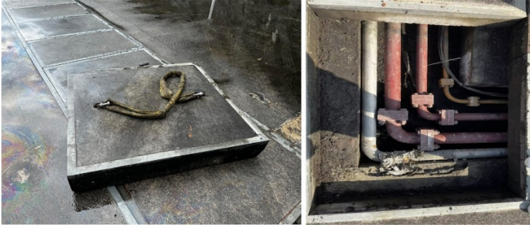
Fig. 1. Oil pipe trench and concrete slab on the lock surface of the Three Gorges ship lock.
