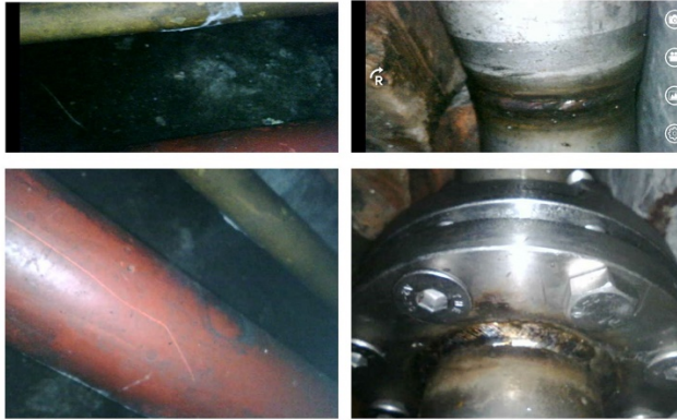
Fig. 12. Field application of industrial endoscope camera.
