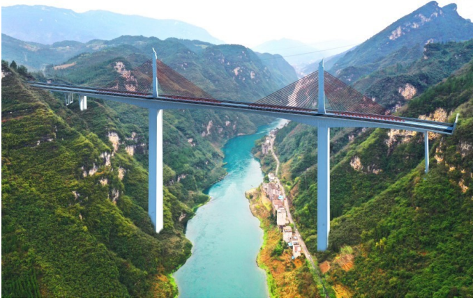
Fig. 1. Overall effect of mozhai wujiang super large bridge
