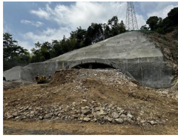
Fig. 1. The entrance section of the left line of the Xiangjianling Tunnel
