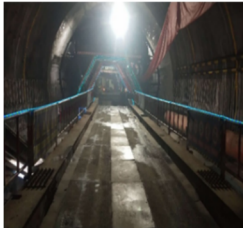
(e) Self-propelled hydraulic inverted arch trestle
