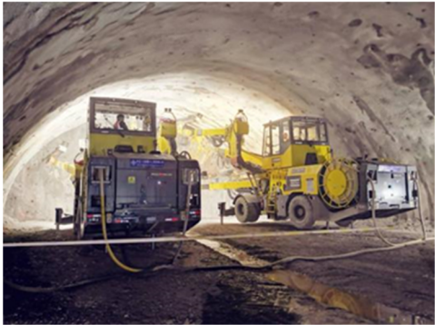
Fig. 4. Simultaneous drilling by two three-arm rock drills.
