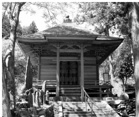
Fig.4. Kannon-dō of Tenyuji temple, restored in 2016 (source: Author)
