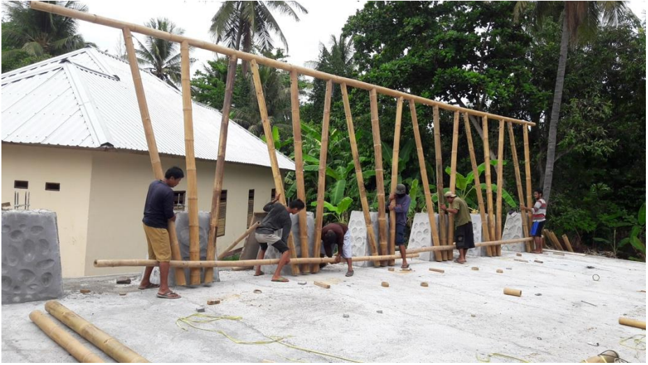
Fig. 8. Erection of the first prefabricated planar module
