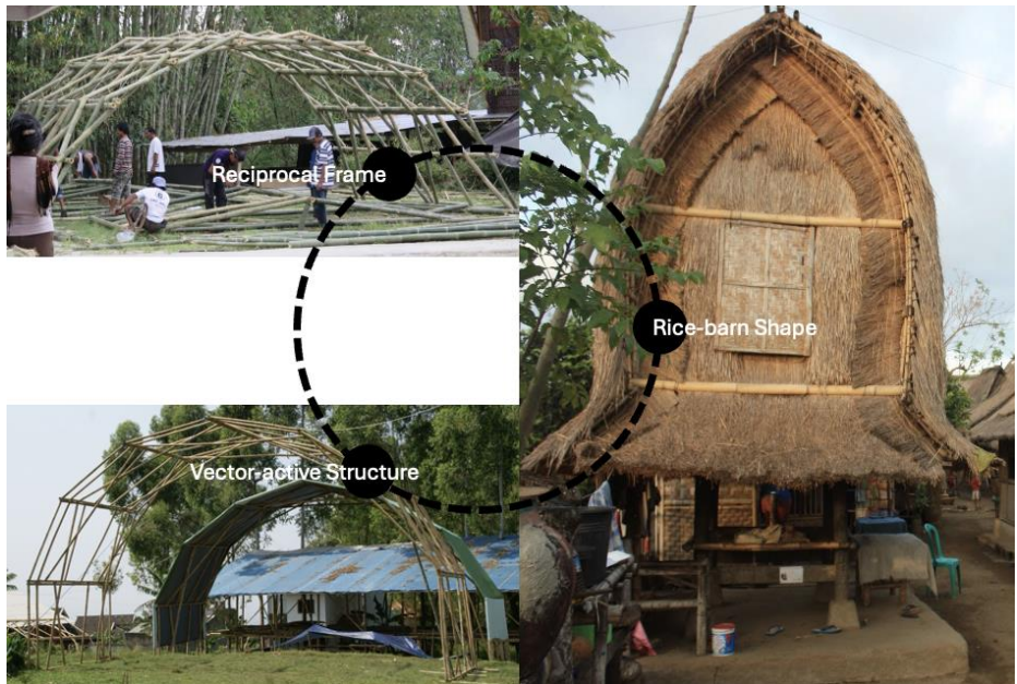
Fig. 1. A Fusion of architectural traditions (rice-barn shape) and structural innovations (reciprocal frame + vector-active structure).
