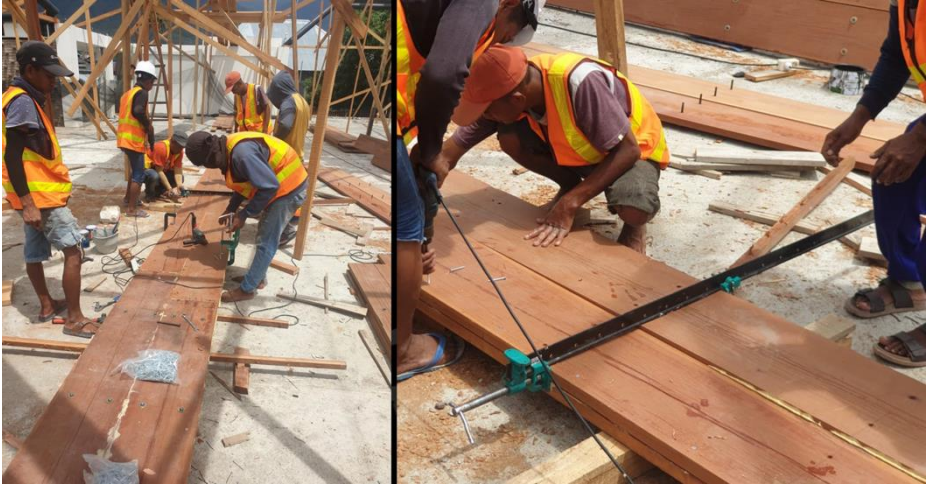
Fig. 11. Manual lamination technique to form main beams
