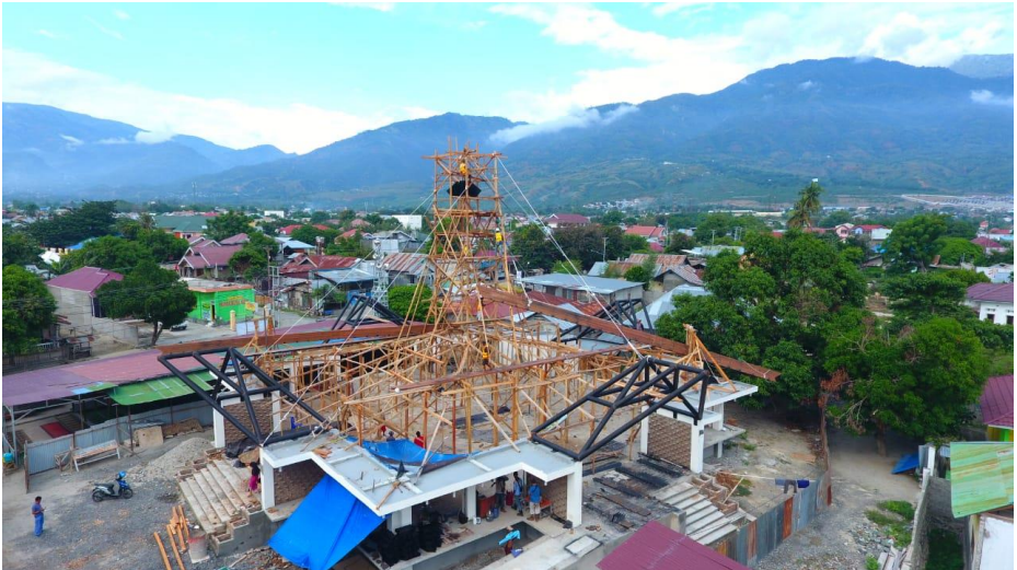
Fig. 12. Erection of main beams using tackles and pulleys
