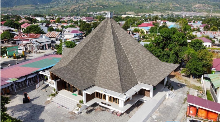
Fig. 13. The appearance of the mosque building from a drone's perspective
