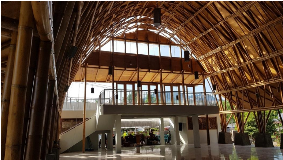
Fig. 10. Interior of the mosque, showing the structural layers of bamboos
